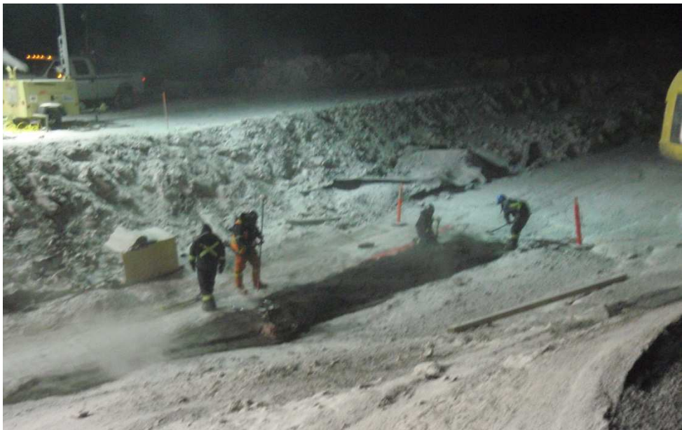
Photo 17: Placing and spreading FCM by hand around the fillet expansion at station 0+60 to 0+70, ~ SW view.
