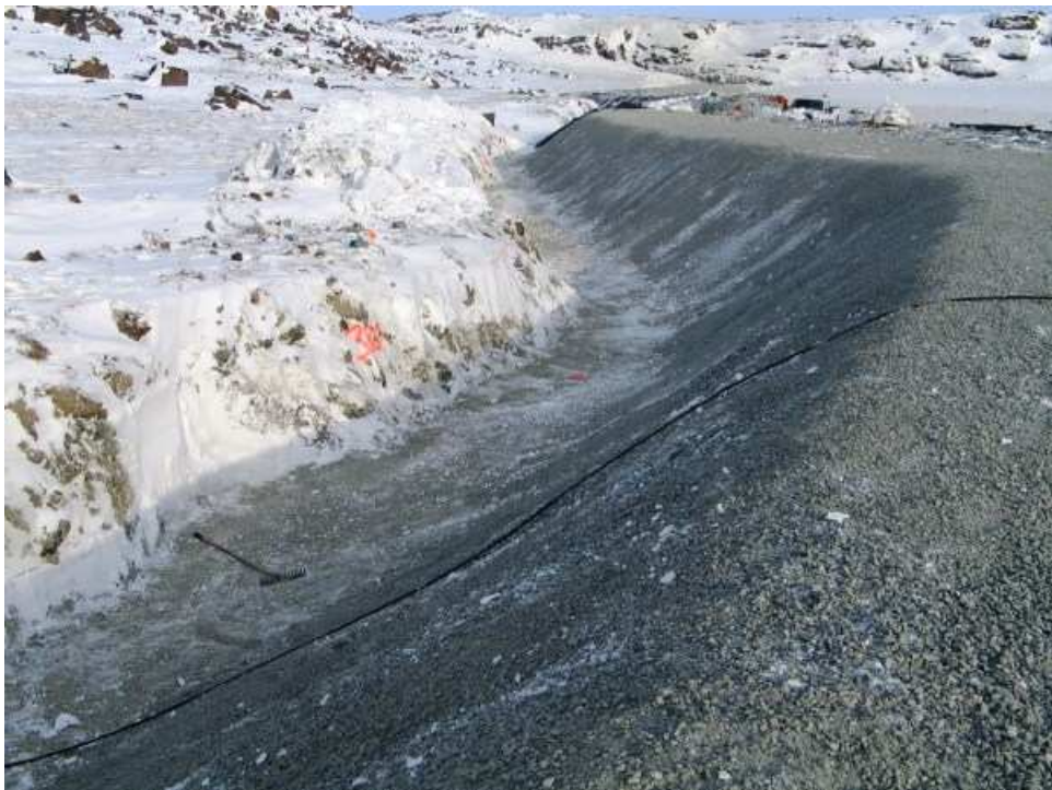
Photo 11: Cleared area ready for geotextile
