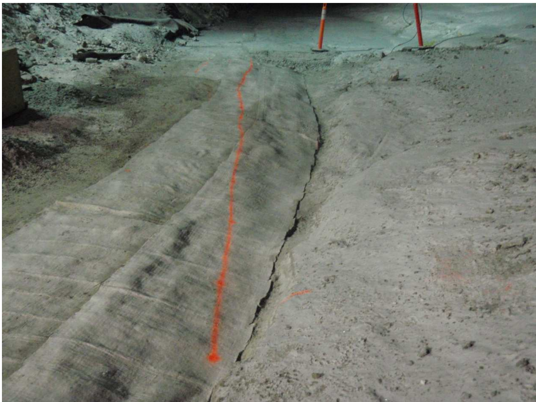
Photo 16: ~WSW view of GCL repairs around the fillet expansion at station 0+60 to 0+70.
