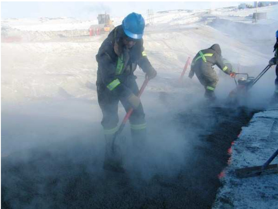
Photo 6: Raking and packing 1st load
