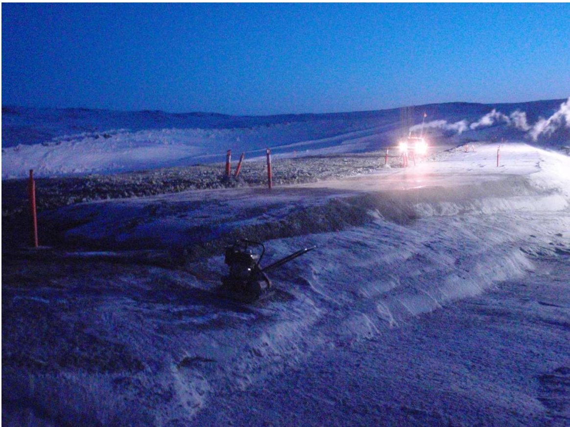
Photo 20: ~N view of core placement around station 0+47 to 0+65. Note plate tamper in foreground that was used to pack the upstream edge.
